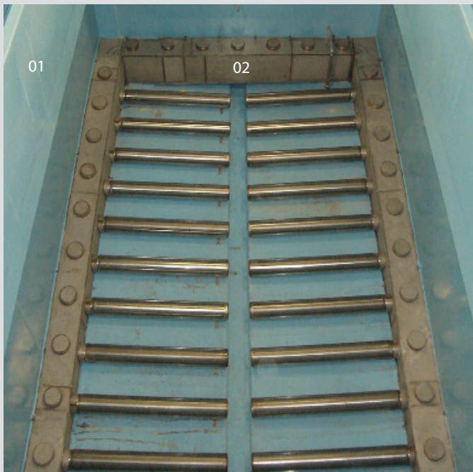
01 Round Triton underdrains with an integral flow distributing manifold 02 Flow distributing manifold 03 Basin with a sloped floor, center eductor and off-center water header
